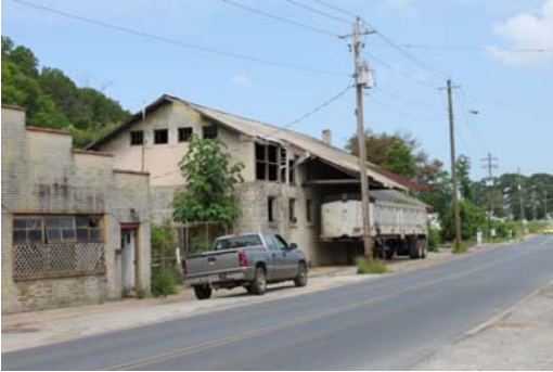
This area contains deteriorating older industrial buildings.
