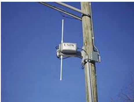
Examples of Wi-Fi using routers deployed outdoors, often on poles
