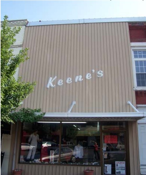
This canopy covers the second story windows
