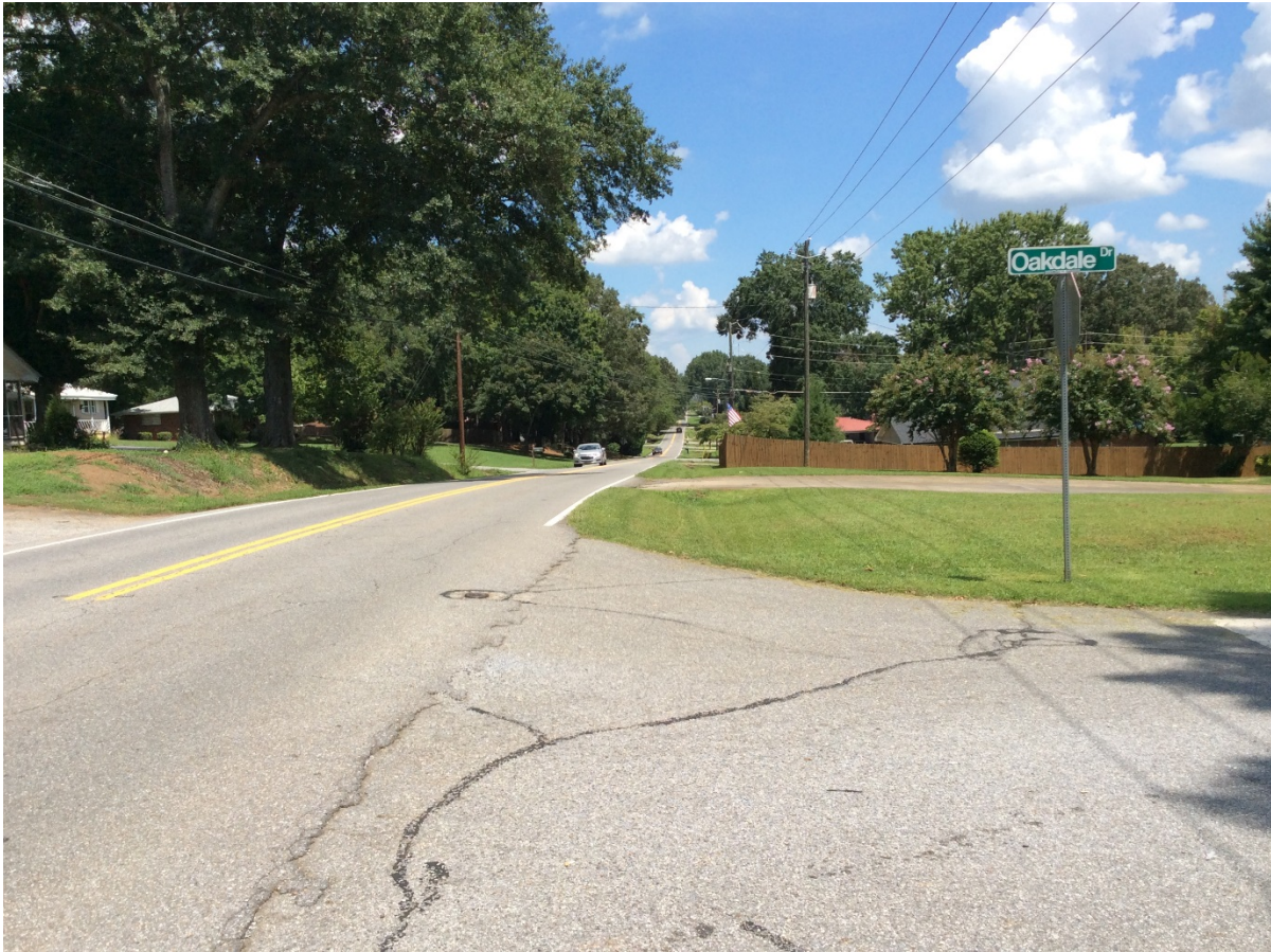
Looking north from intersection of Oakdale Drive and Grassdale Road
